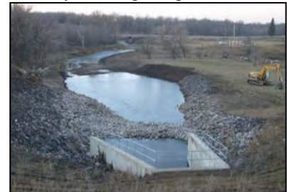
Looking downstream from outlet structure
