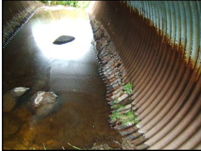
Rusted out culvert under a township road in branch 13 of JD 72 that had to be replaced
