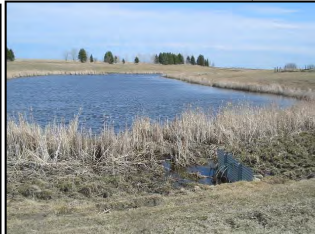
Thibert Dam, Red Lake County
