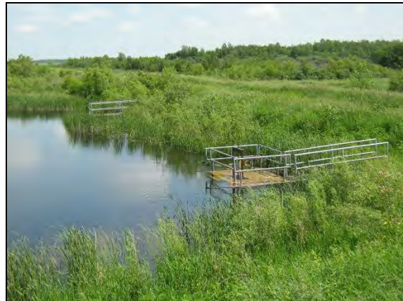
June 27, 2014 – Pool elev. – 1174.8 (deck of structure was submerged)
