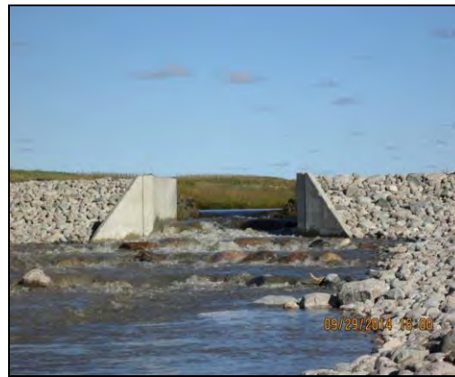
NRCS drop structure after construction
