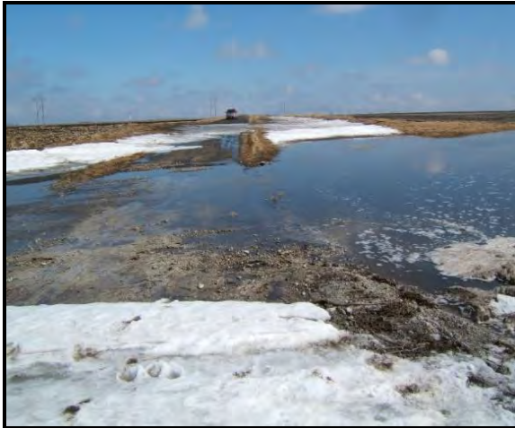
Spring runoff water starting to overtop road
