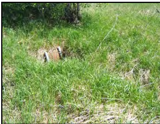
Plugged side water inlet pipe before project
