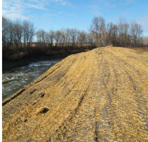
Slope seeded and mulched
