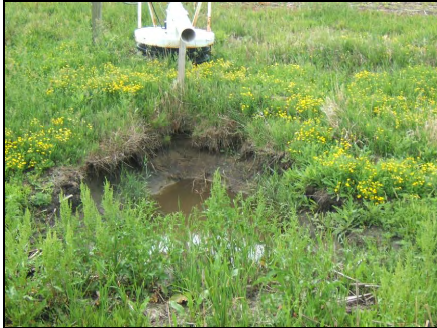
No erosion control at the outlet of a tile pump
