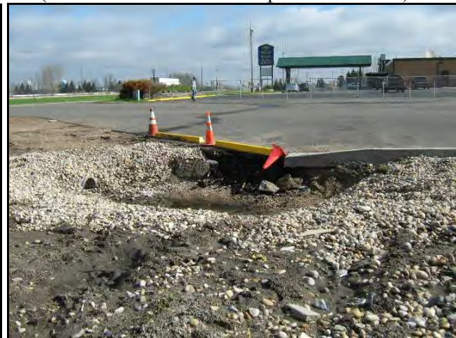
Grand Stay Motel, Thief River Falls (culvert extension with 'drop-inlet' installed)
