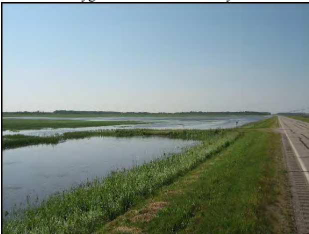
North of Grygla after 4.3 in. rain-July 2014
