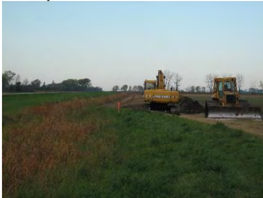
Inlet Channel – looking west – approx. ½ mile was widened to enhance flow conveyance and excavated material was used to construct an adjacent berm.
