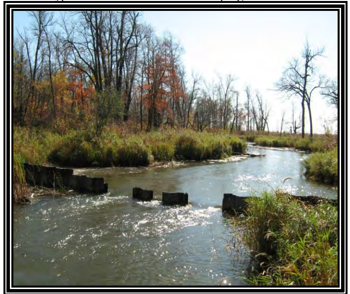
Typical Fall Drawdown with Stoplogs Removed
