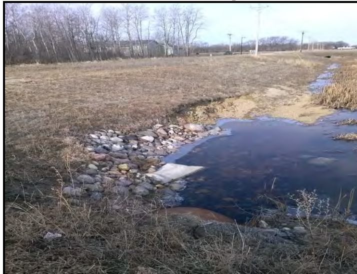
Erosion area caused by a storm water outlet
