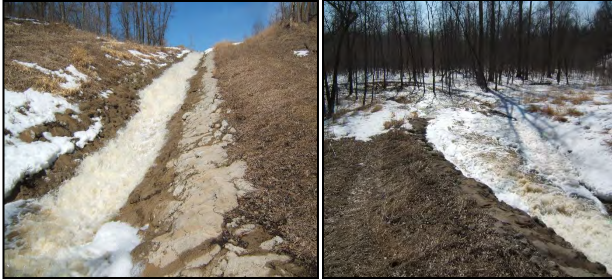
Spring runoff water flowing down the rock chute and into the plunge pool on RLWD Ditch 10 (Project #161)
