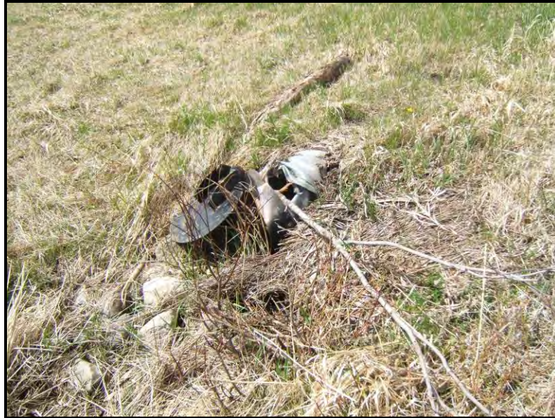
Side inlet pipe and trap destroyed by a mower
