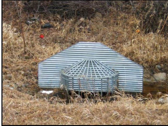
Cleaned trash rack
