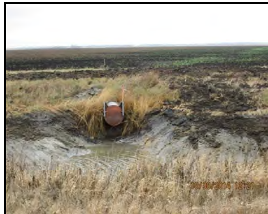
Cleaned side water inlet pipe after project
