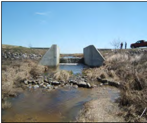
NRCS drop structure before construction
