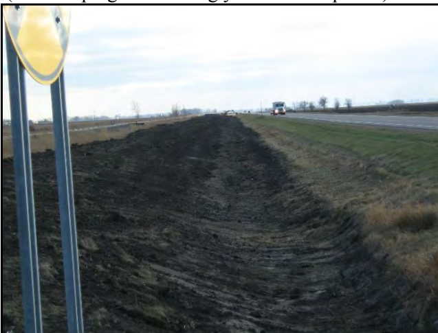
Ditch Cleaning. U.S. Hwy. #75 near Euclid (final shaping and seeding yet to be completed)
