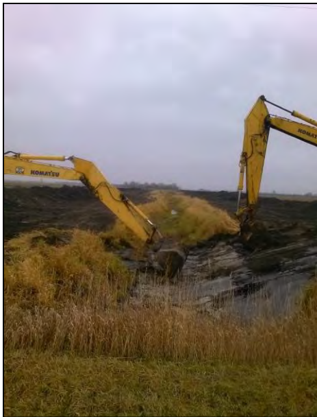
Berm Stripped, Starting Channel profile excavation.
