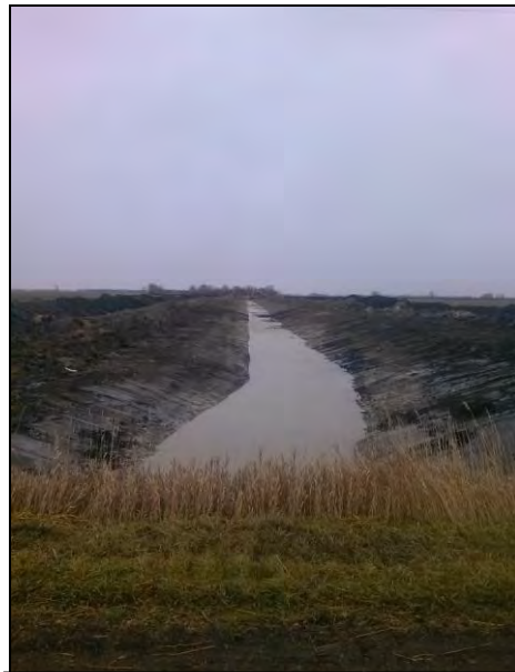
Channel profile excavation complete. Berm shaping and black soil needed.
