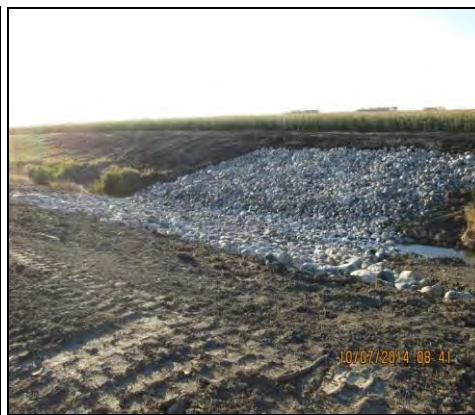
One of nine rock checks installed after project
