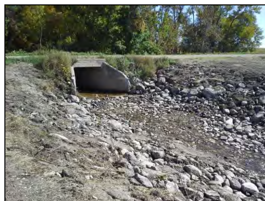
Box culvert after project
