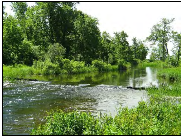
Pine Lake Dam-Lake elevation approx. 1.2 ft. above summer level-June 2014
