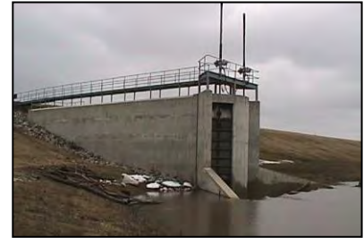
Principal outlet structure hydraulic gate operation
