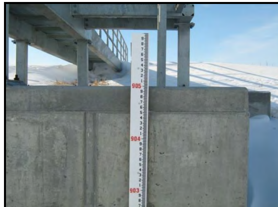
Typical staff gage at structure
